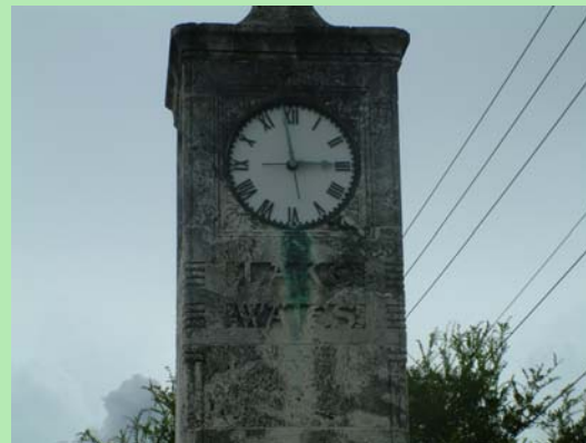
Lake Wales received its unique clock tower in 1931. The clock tower was a gift to the City of Lake Wales from Misses Sara E. and Emma Y. Kolb. The core of the tower is brick, with a coquina façade.
