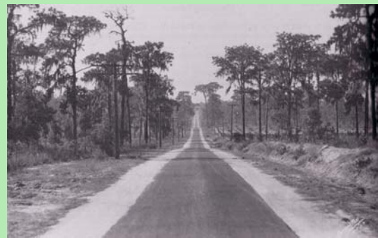
Scenic Highway, asphalt lane with clay shoulders (Source: Crooked Lake – Babson Park Rediscovered)
