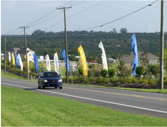
Figure 9. New development along SR 17 – North Lake Wales
