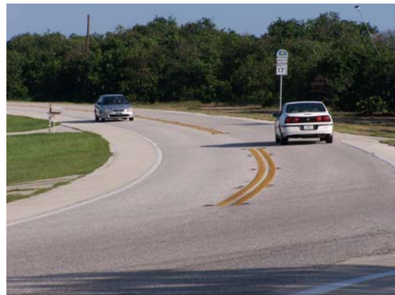
Figure 2. SR 17 curve near Highland Park
